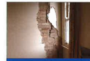
Reconnecting Separated Walls
