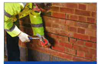
Creating Load Bearing Masonry Beams
