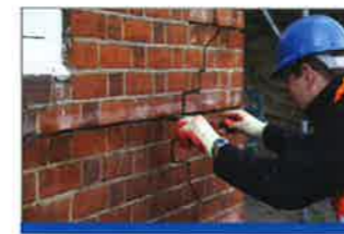
Crack Stitching
