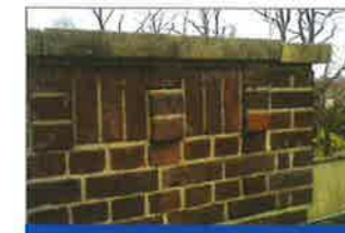
Securing Parapet Walls
