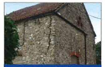
Stabilising Rubble-Filled Walls
