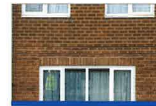
Lintel Repair & Creation
