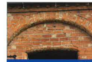
Repairing Masonry Arches
