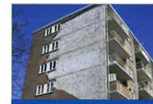
Replacing Failed or Omitted Wall Ties
